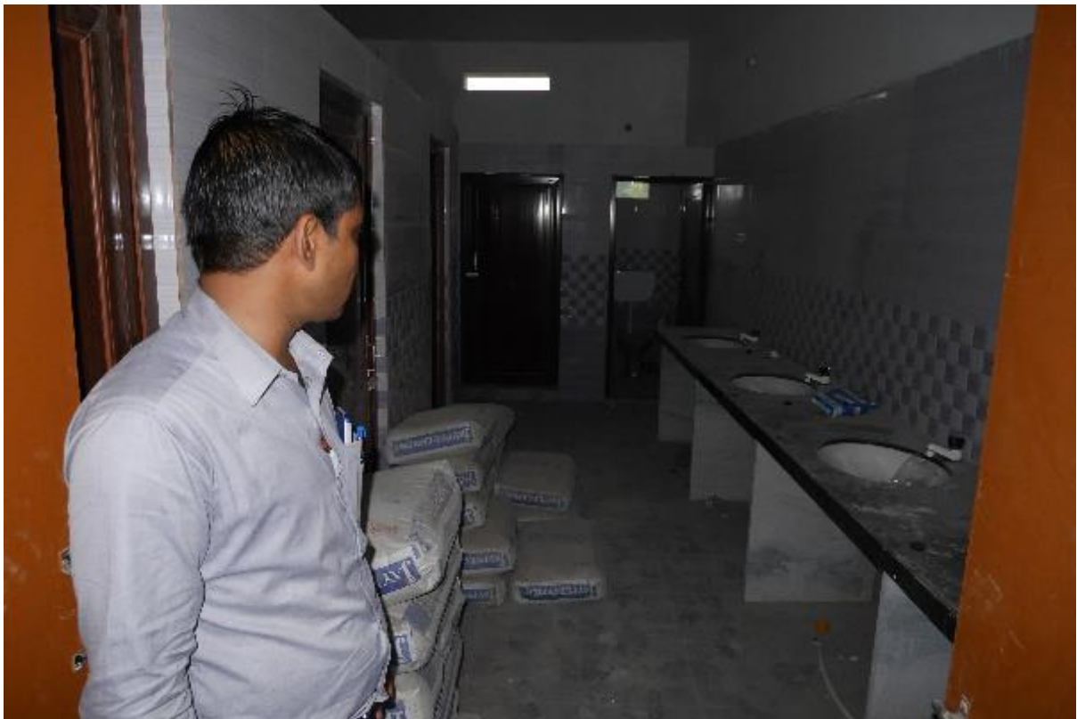
The patients' future washroom is better than some army toilets.
